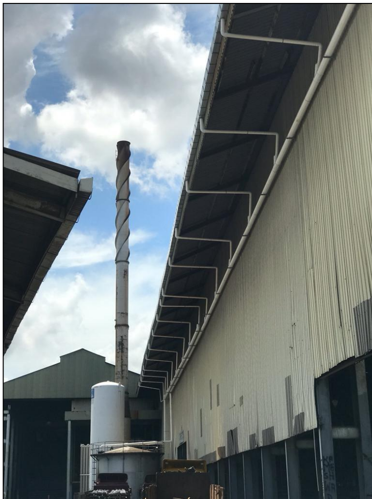
Rainwater harvesting system being installed at the Petaling Jaya plant
